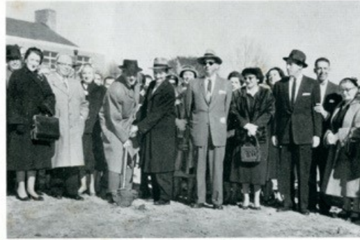
Ground Breaking Ceremonies February 17, 1957. Mayor E. J. Evans and Rabbi Louis Tuchman are shown in the center of the picture breaking ground.
